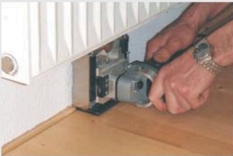
Cutting expansion joints under radiators
