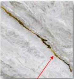
局部实拍 Detail in part
