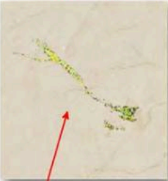
局部实拍 Detail in part
