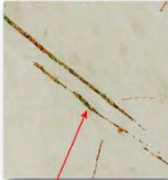
局部实拍 Detail in part
